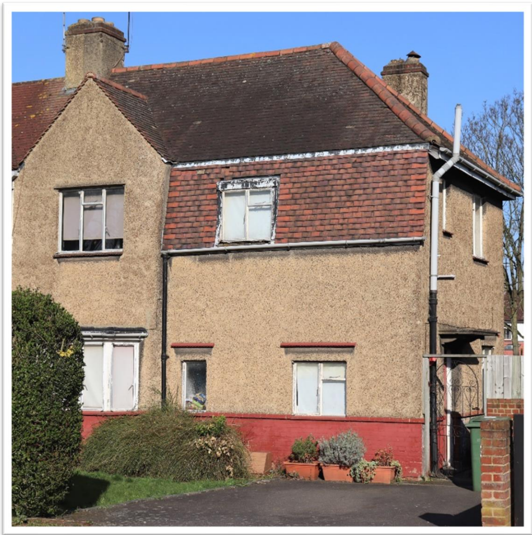
Figure 5. Original features: tiled mansard roof over roughcast rendered walls with metal casement windows.
