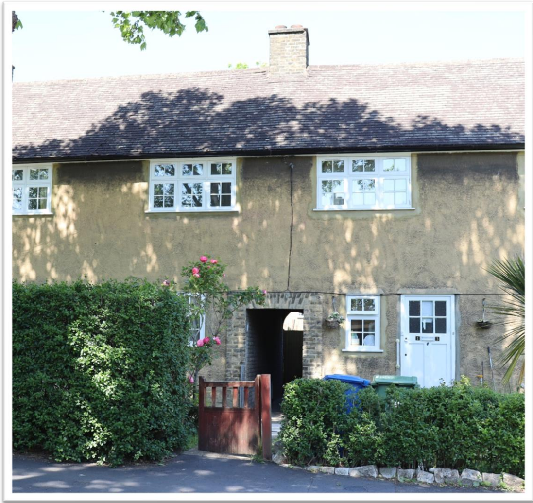
Figure 13. Part rendered walls.
